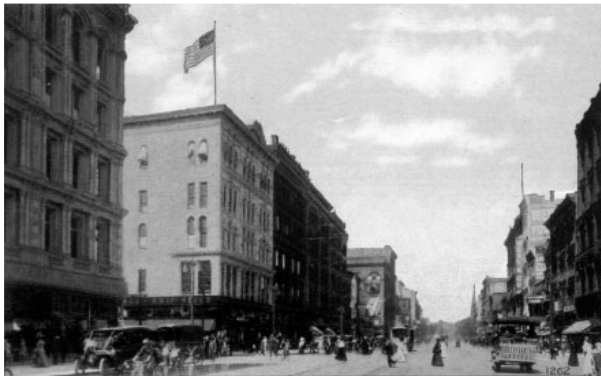
Woodward and State was a busy intersection in 1917. Author's collection.
