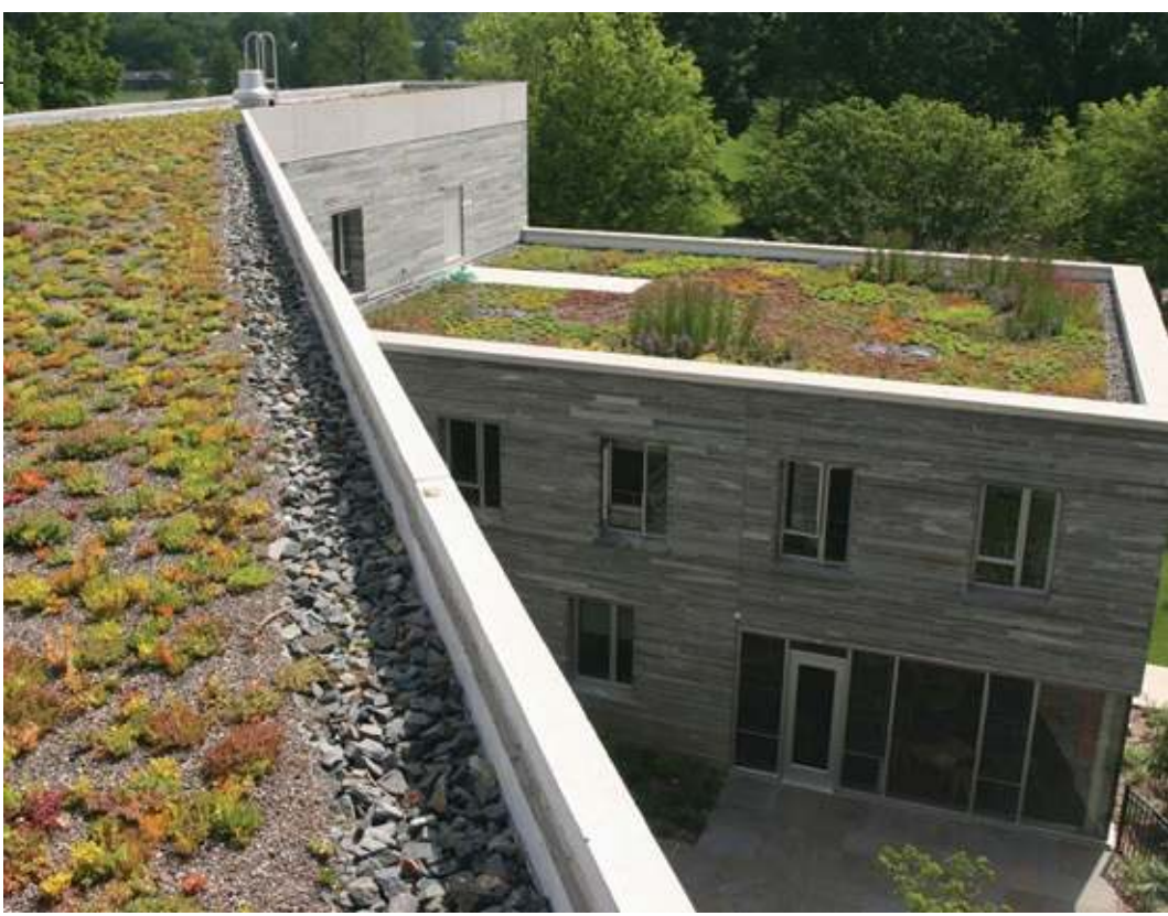
Green roofs are increasingly popular on college campuses. This dormitory at Swarthmore College has green roofs on two levels, one of which is visible from inside the building.
