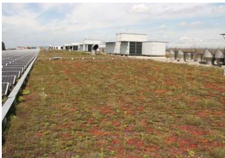
Extensive green roofs, especially when installed on a wide scale, provide a range of benefits including stormwater management.
