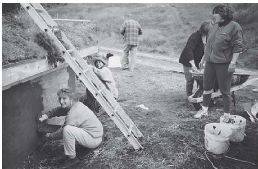
Happy crew at work during a straw bale workshop.
