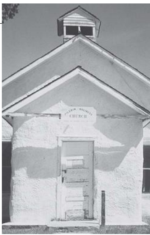
The Pilgrim Holiness Church in Arthur, Nebraska, built by the congregation with donated rye-straw bales.
