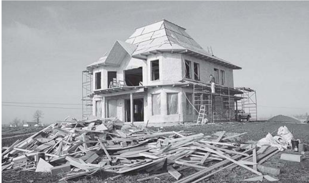
A small pile of recyclable materials is often all that is left over after construction of a straw bale house.
