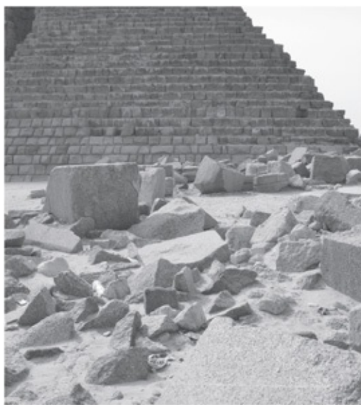
Fig. 1.1. Vast amounts of granite rubble surround Giza’s third pyramid. Notice that some of the pyramid’s granite casing stones remain in place.
